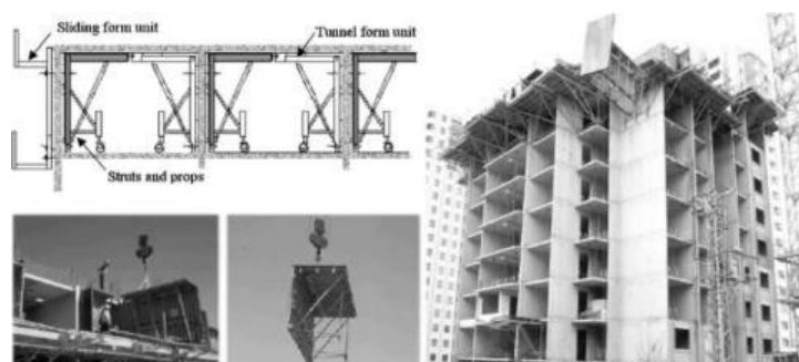
Figure 14.15: Tunnel formwork technique
