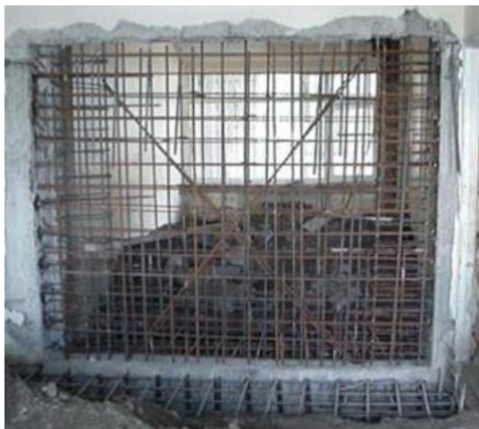
Figure 14.7: Additional Shear Wall
